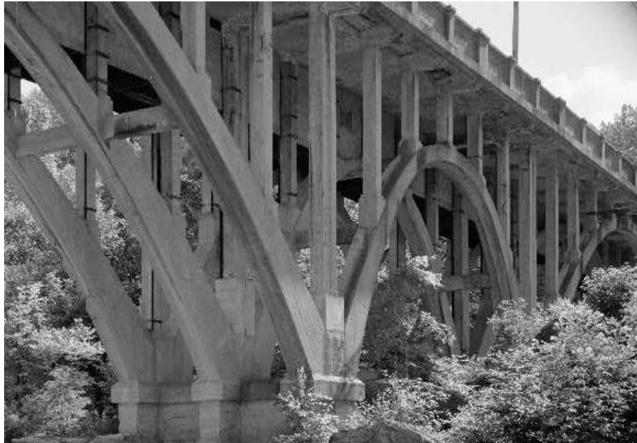
Figure 4.5 – Photograph of the Woronoco Bridge in which the spandrel columns are visibly enlarged where they are connected to the arch ribs (courtesy of HAER/LOC).
