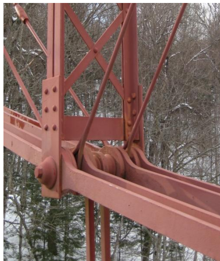
Figure 8.2 – Lower chord connection at Bardwell's Ferry Bridge (courtesy of HAER/Library of Congress).
