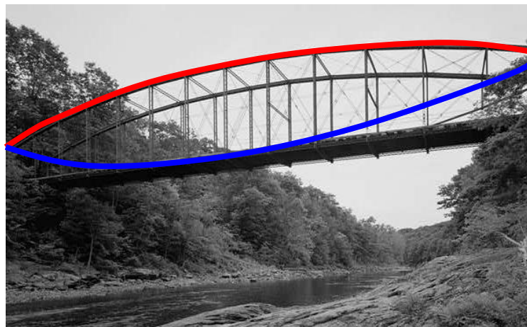
Figure 7.1 – Bardwell's Ferry Bridge illustrates the two structural forms integrated in lenticular bridges: the arch (red) and suspension cable (blue) (photograph courtesy of HAER/Library of Congress).
