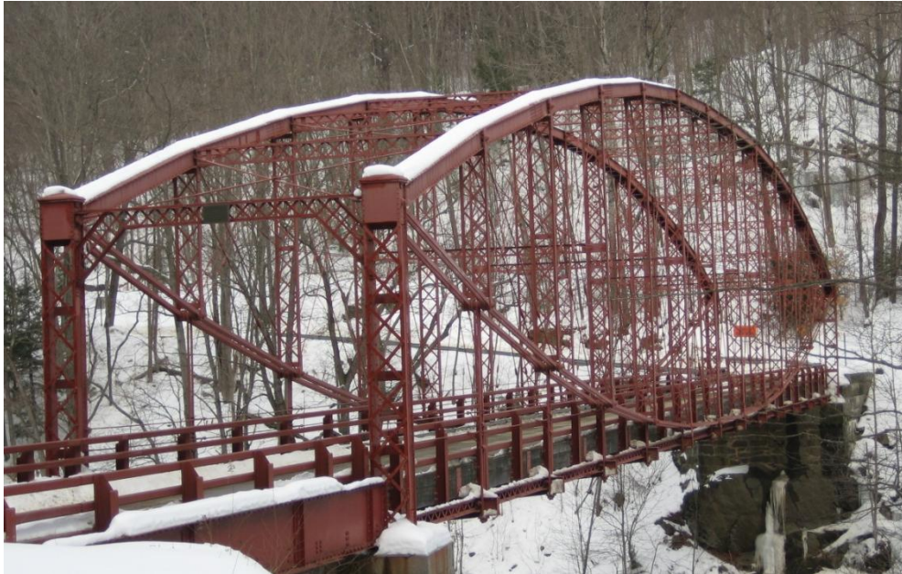
Figure 8.1 – Photograph of Bardwell's Ferry Bridge.
