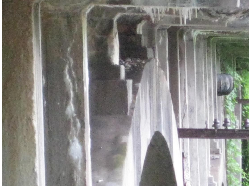
Figure 4.7b –Lack of cracking between the spandrel columns and the arch (photograph taken in June 2009).
